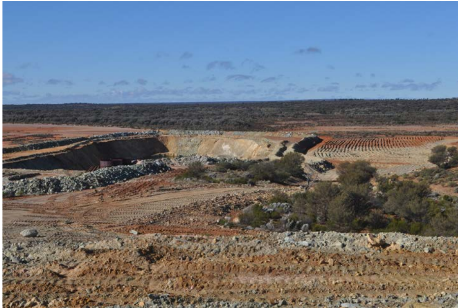
Photo of the Devon Gold Project showing rehabilitation work
